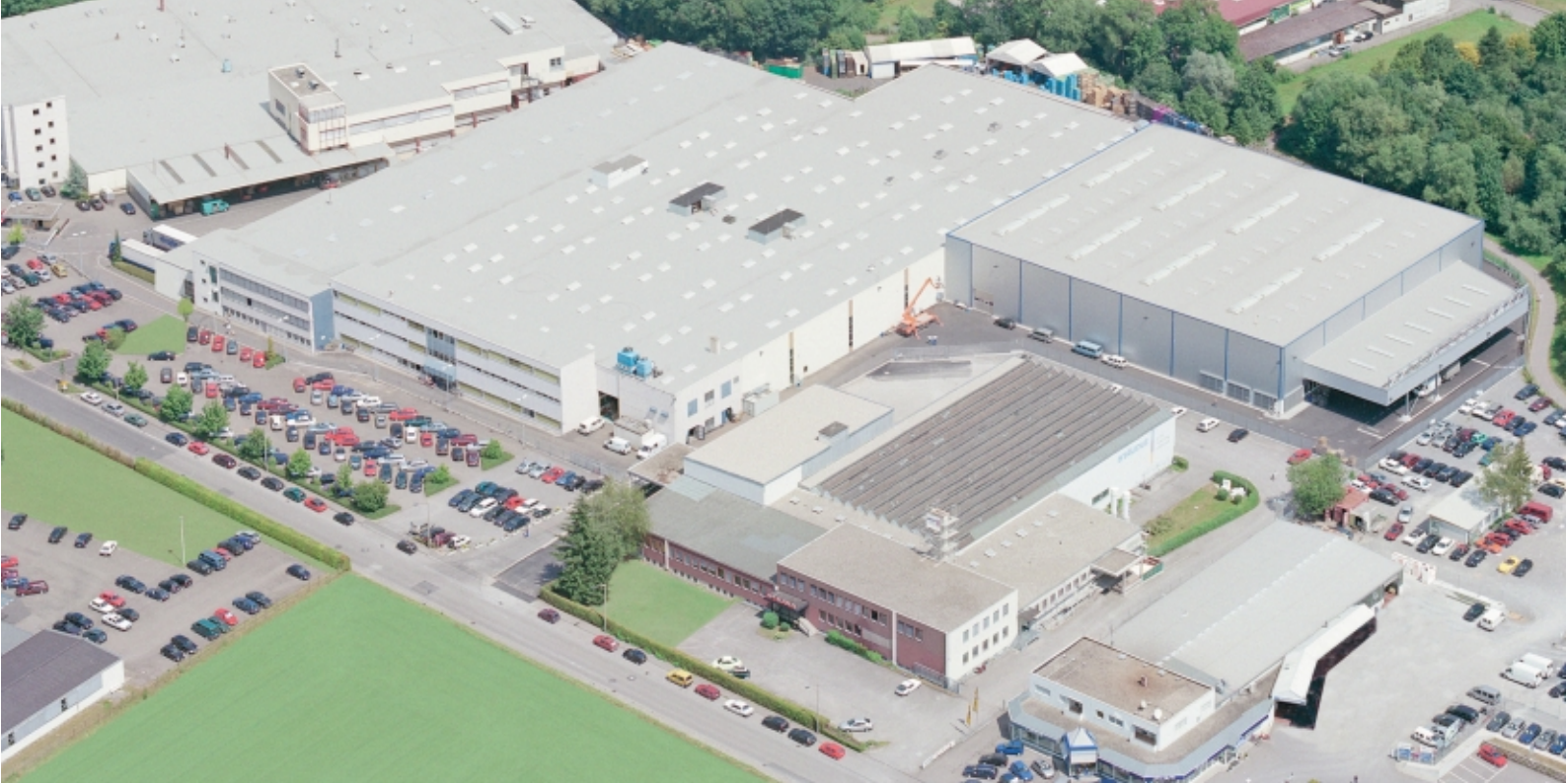
MAHLE Industrial Filters, Öhringen plant
